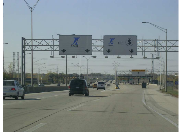
Figure 6: Drivers with special transmitters can pay tolls without stopping (i.e. breaking the connection)
